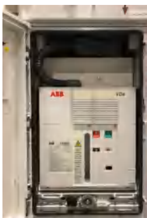
Figure 3-1 Circuit-breaker compartment, open. Withdrawal part in the disconnected position
