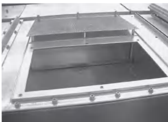
Figure 56 Openings on top of the gas duct
