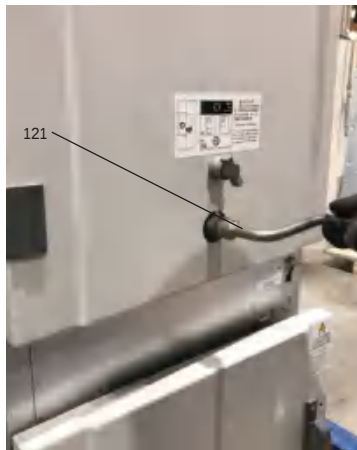
Figure 63 Movement of the withdrawable part between the test/ disconnected position and the service position: clockwise up to the stop for service position and anticlockwise for the test/disconnected position
