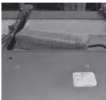
Figure 49 Transport position of antiferro-resonant resistor
