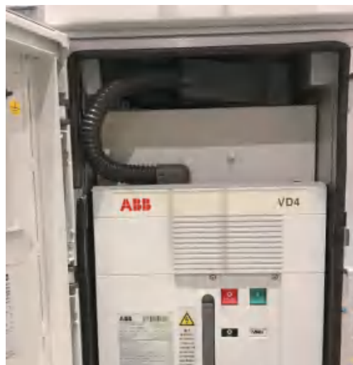
Figure 61 The control wiring plug connector is blocked to prevent disconnection with the withdrawable part in the service position
