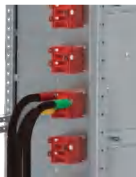
Form3b cable connection without separation
